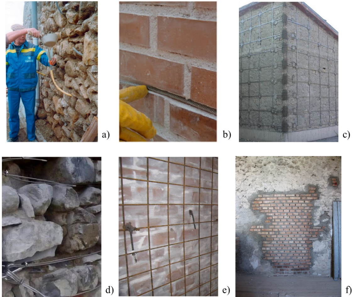
Figure 2.8 Some interventions to increase the masonry strength: a) Injection of binder mixtures; b) Re-pointing of the joints; c) Tie rods opposing to both deformation and disconnection of wall panels ; d) Insertion of stainless steel cords in the mortar joints ; e) Reinforced concrete; f) “cuci-scuci”.
