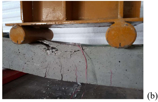
Figure 17 – (a) View of beam B0 at failure; (b) detail of cracking with detachment of compressive concrete.
