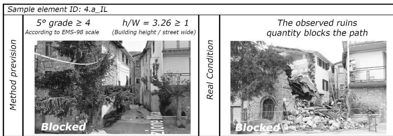
Figure 2 Comparison between the Observed macroseismic damages-based approach prevision and real conditions of path blockage for a building in the sample (Element ID code: 4.a_IL in Appendix B ): the path is effectively blocked because the observed damage is higher than the 4 th grade and the ratio between building height and street width is higher than 1.
