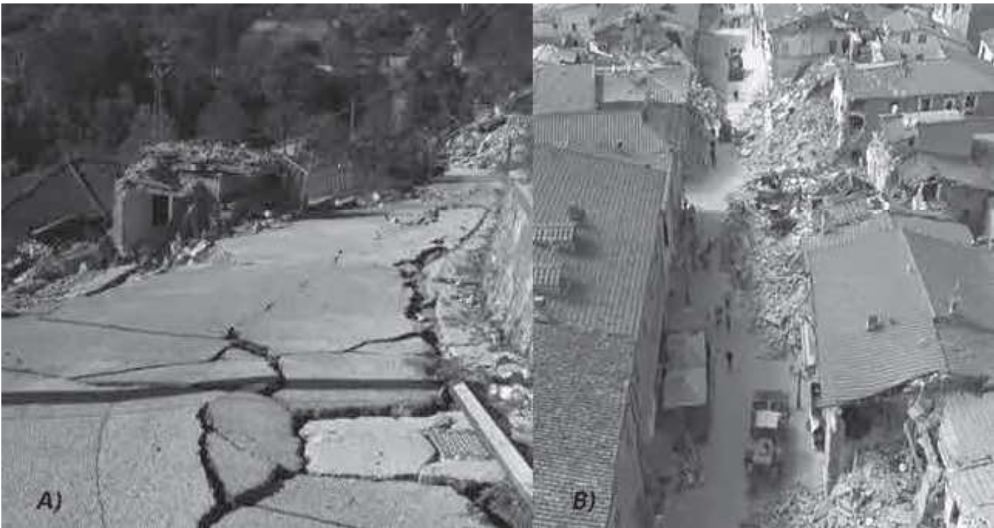
1223 1224 Figure 2 Urban scenario damages in the Central Italy seismic sequence in 2016: A) street pavement cracking due to unstable slopes 1225 and landslides-induced effects (Intrinsic vulnerability); B) an aerial view of Amatrice (RI, Italy) main street, that is partially blocked by 1226 ruins formation provoked by buildings collapse; debris impeded rescuers' interventions (Extrinsic vulnerability). Video frames by Corpo 1227 Nazionale dei Vigili del Fuoco http://www.vigilfuoco.tv/ (last access 2018/04/17). 1228 1229
