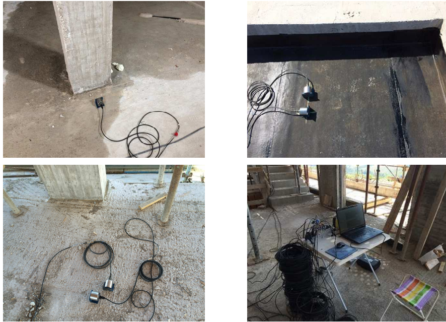
Figure 1.12 Arrangement of the accelerometers on Building 1.
