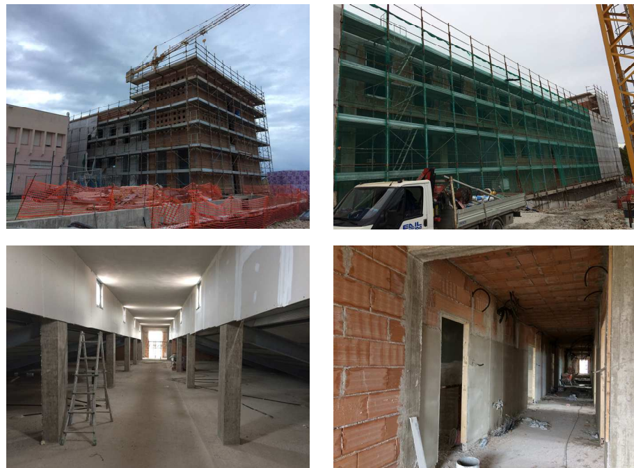
Figure 1.15 Building 1: construction process on November 7, 2016.
