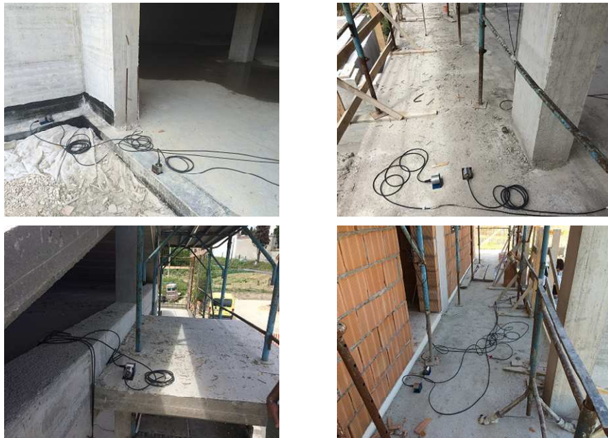
Figure 1.13 Arrangement of the accelerometers on Building 2.
