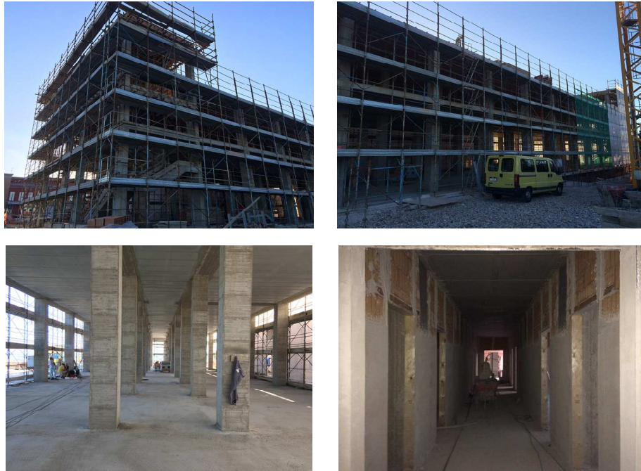
Figure 1.14 Building 1: construction process on August 25, 2016.
