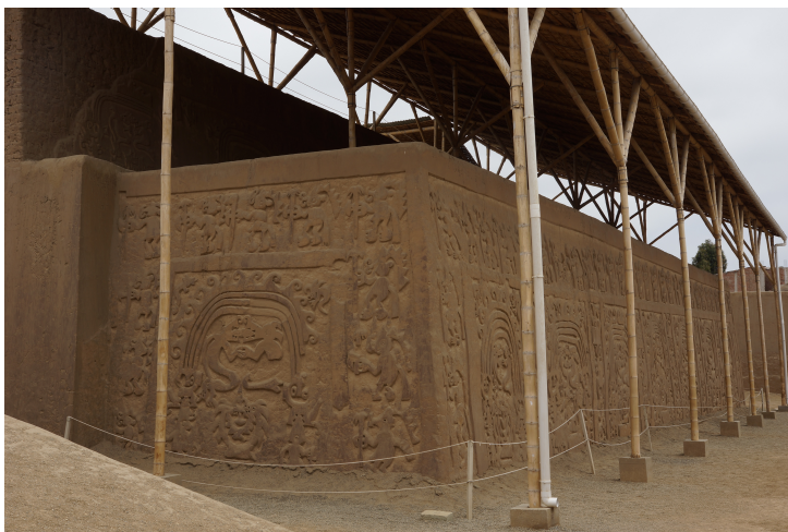
Figure 3.11: Large coverings that spoil the visual impact of the building and decorations.
