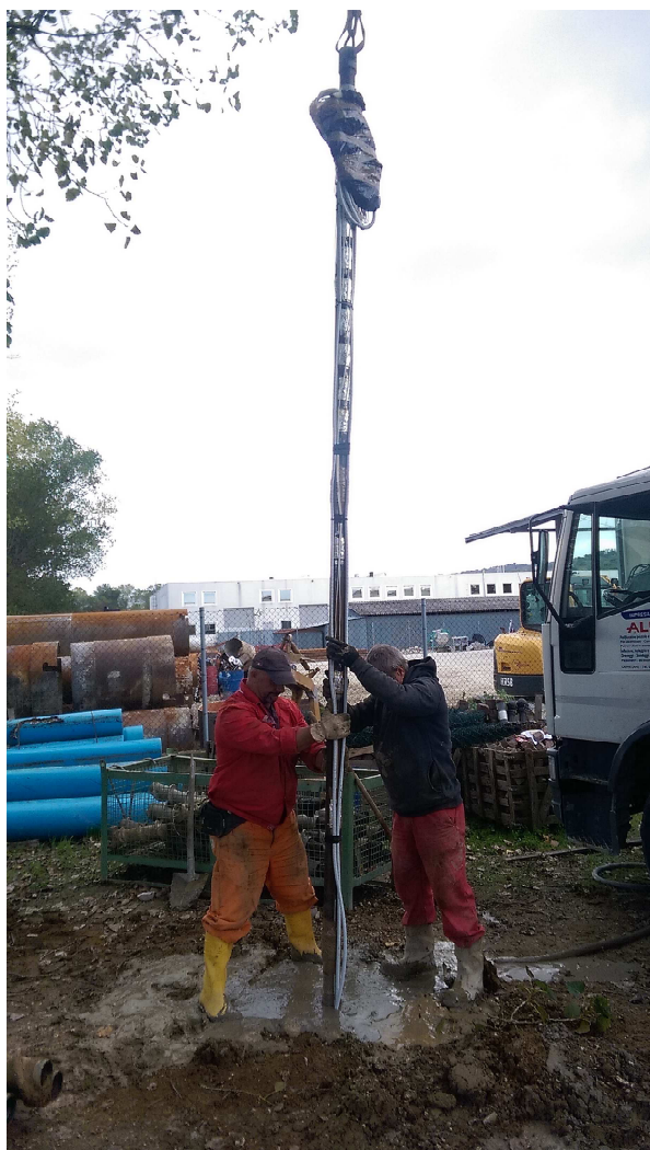
Figure 4-8 Insertion of an instrumented micropile into a grouted borehole
