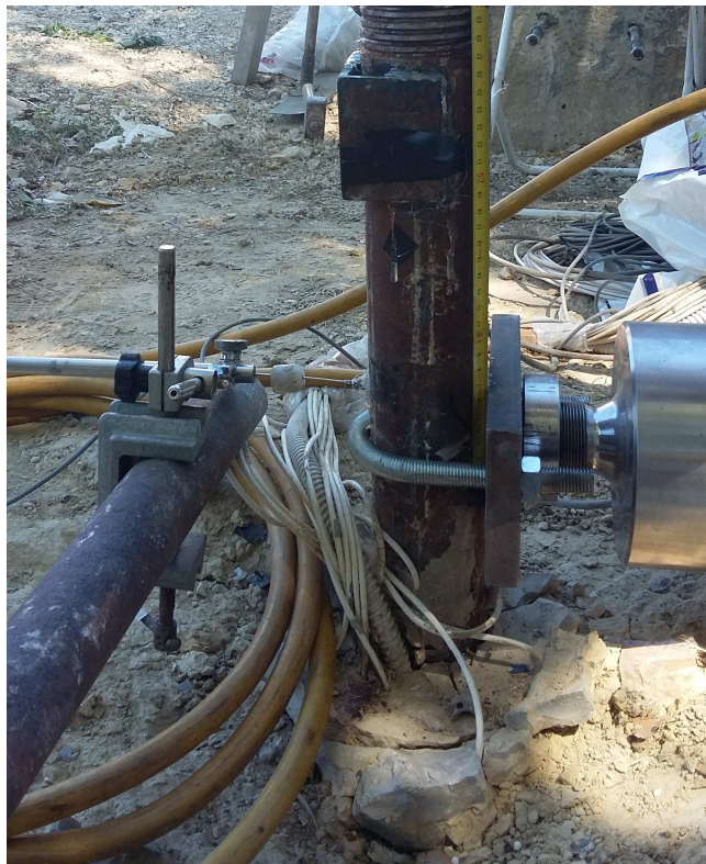
Figure 4-34 Details of the coupling between the load cell and pile P1
