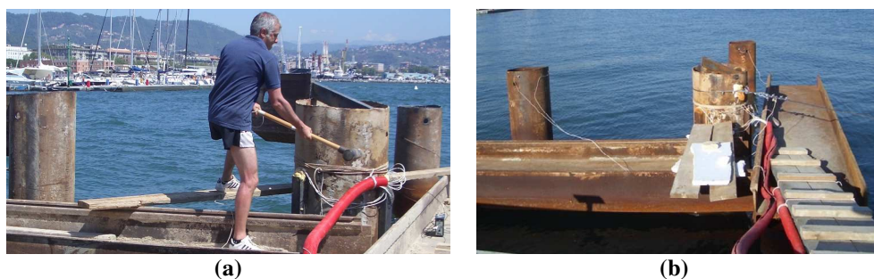
Figure 3-8 Impact load tests (a) and free vibration tests (b) performed by Dezi et al (2012, 2013, 2016) on three near-shore steel pipe piles vibro-driven into soft marine clay
