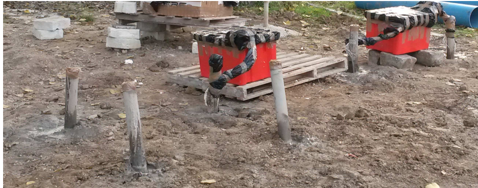
Figure 4-11 View of micropiles after high pressure injections
