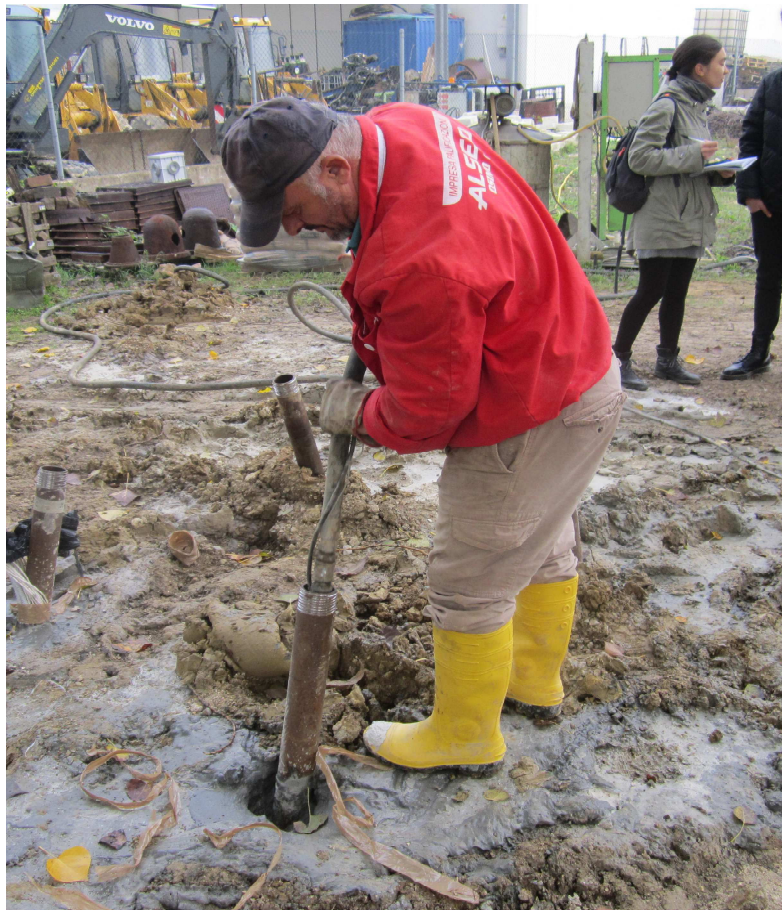
Figure 4-10 Execution of high pressure injections
