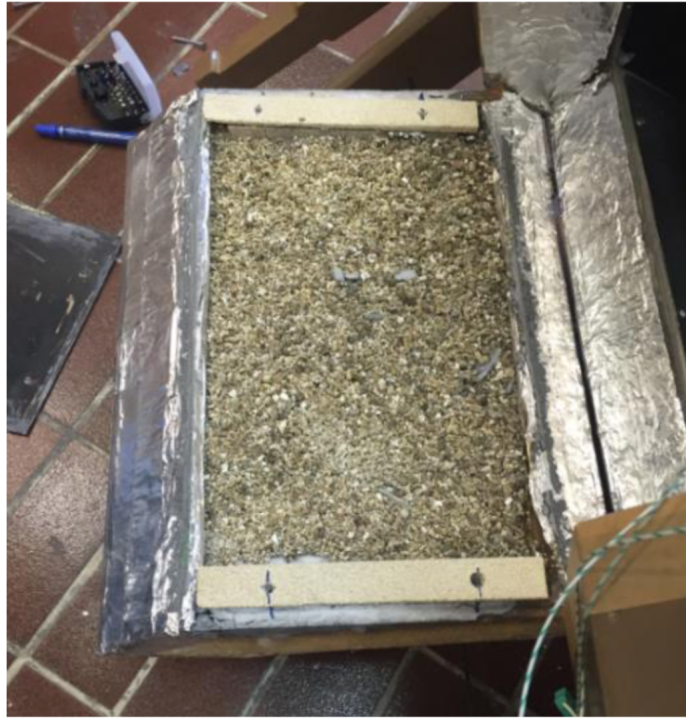
Figure 4.9: Vermiculite inserted in the small door cavity.
