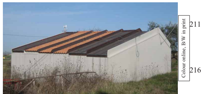
Figure 1. South view of the experimental building near Ancona (Italy).
